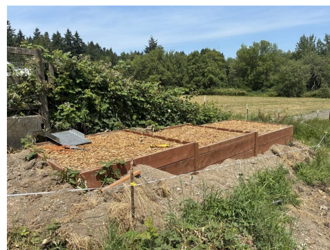
A Denitrifying Bioreactor (above) uses carbon to manage nitrogen
