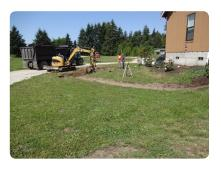
Raingarden #3 is prepared, according to specifications. Next, engineered soils will fill this area, prior to the planting phase. Photo: Karin Strelioff
