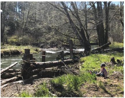
These engineered log jams are carefully designed to withstand high flow events and allow for safe recreational river use!
