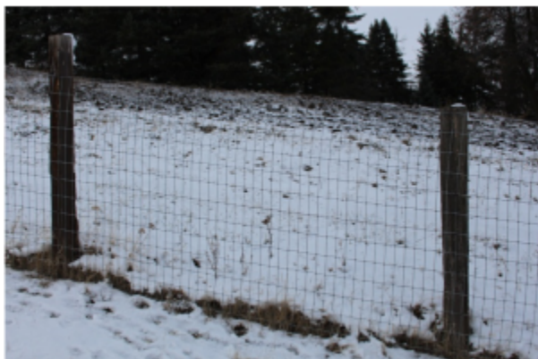
Figure 4. Woven wire fencing with small openings. This style of fence is frequently preferred by sheep and goat owners. Photo by Mark Heitstuman.
